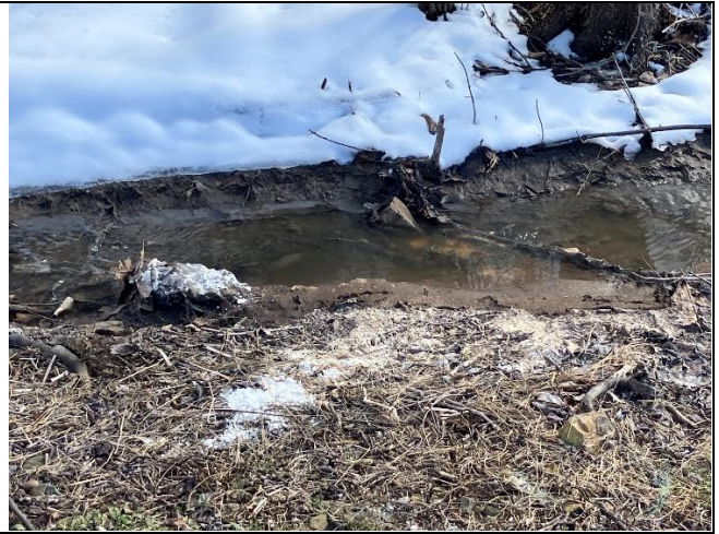
2 – Ditch next to Equalization Basin conveys overflowed wastewater to the wooded area downgradient of the basin.
